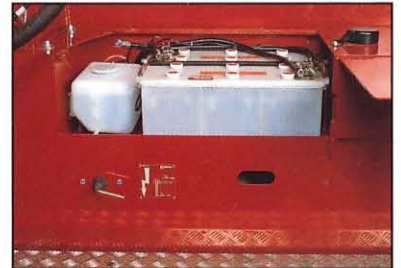
The battery box with mains switch is located on the left-hand side of the truck.
